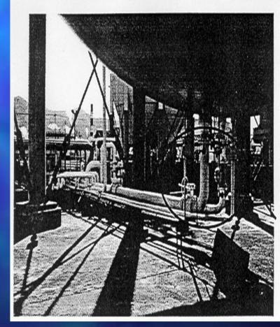
Flanges, valves, fittings and piping are not protected by fireproofing nor water spray systems
