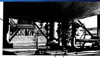
Numerous gaskets, bolted flanged connections, and control valves are directly under the tank.
