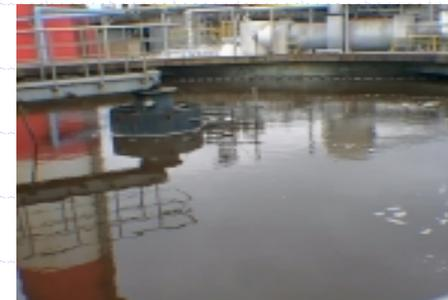
**Advanced ASP: nutrients are removed by altering oxic and anoxic bioreactor condition**
