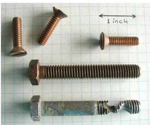
Crevice corrosion of a bolt
